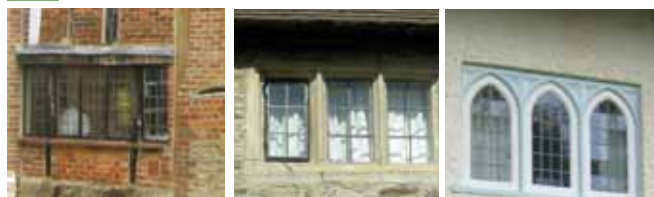
287 Casement windows with leaded lights - ranging from timber to stone. Designs dependant on the period. Occur from Medieval to inter-war period.
