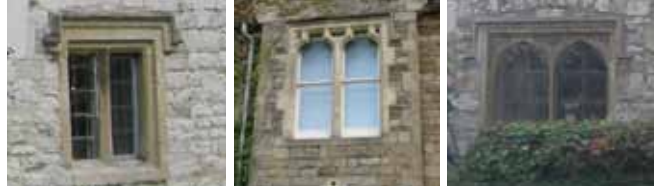
286 A variety of stone-mullioned and often transomed windows. A range of head designs from square, rounded and cusped. Windows are typical from Medieval to Victorian periods
