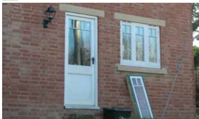
291 When replacing windows it is important to undertake a like for like replacement - as seen here.
