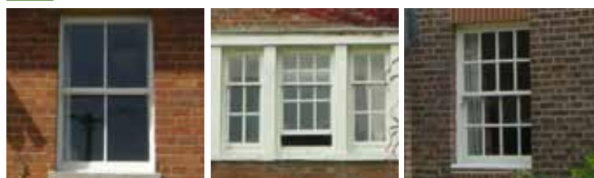
289 Sliding sash - designs with a taller vertical emphasis. Ranging from 4 to 16 or more lights. Occur from Georgian to Edwardian periods.
