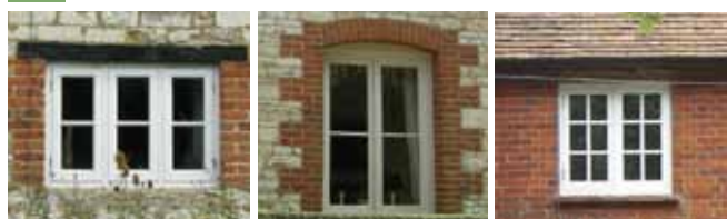
288 Timber cottage casements painted (see Appendix D for colours). Range of 2, 4 and up to 12 light casements. Occur from late Medieval to present.
