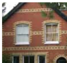
Decorative bands of brickwork are usually found on Victorian properties and are difficult to replicate successfully on new dwellings. On traditional extensions however, the pattern should be continued.
