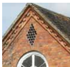
Dentil courses and dentilation around the gable where there is a regular pattern of projecting headers with a projecting course of stretchers above and below. Dog toothing is also found, brick projects at a 45° angle to give pointed appearance
