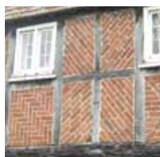
Herringbone patterns are often found in medieval timber framed properties and modern copies. They can take on a number of forms such as vertical, horizontal or basketweave. Sometimes a mix of forms can be seen on the same property
