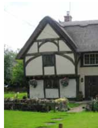
323 Square panelling, with tension braces. A jettied first floor projects over
