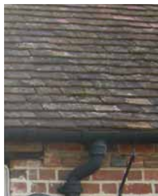
313 Traditional refurbished metal guttering
