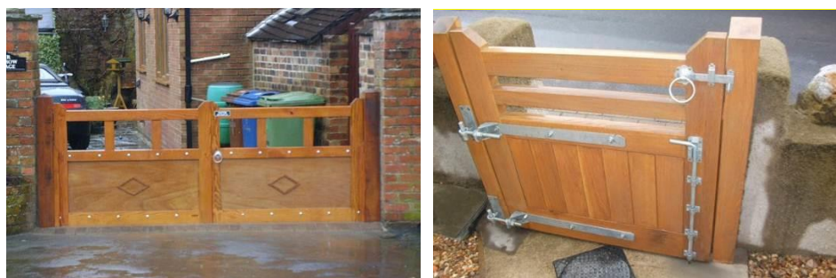
Figure 6-5 Example of flood gates
