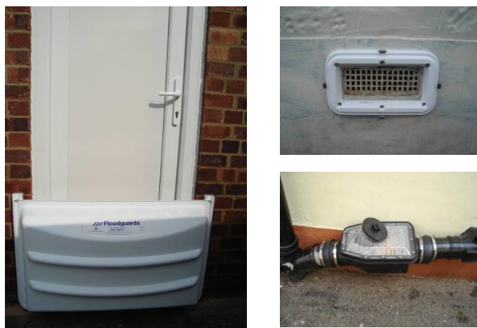
Figure 6-5 Example of flood gates
