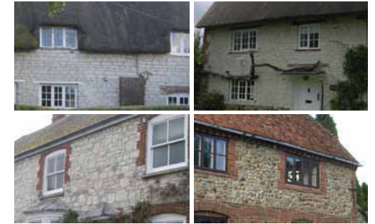
180 Examples of coursed chalk block and uncoursed chalk and sarsen stone construction
