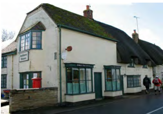
Figure 3.9: Former Post Office - this facility has now been accommodated part-time in the Rose and Crown
