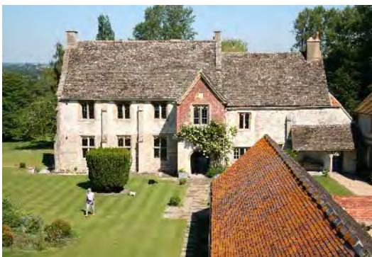
Figure 7.10: Grade II Manor House
