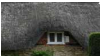
38 Typical thatched roof with dormer
