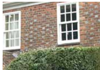
155 Berkshire orange facing brick with burnt or blue headers
