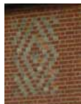
138 Berkshire orange brick with a variety of features including: blue headers and string course, buff detailing, diaper work and dentil and bottle work
