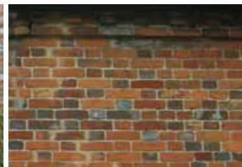
155 Berkshire orange facing brick with burnt or blue headers
