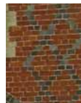
138 Berkshire orange brick with a variety of features including: blue headers and string course, buff detailing, diaper work and dentil and bottle work
