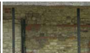
197 Uncoursed chalk with brick repairs
