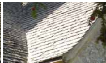
101 Traditional and modern replacement stone slates
