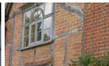
138 Berkshire orange brick with a variety of features including: blue headers and string course, buff detailing, diaper work and dentil and bottle work
