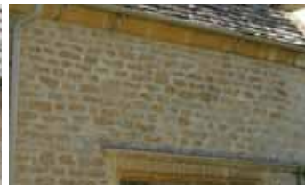
96 Light Corallian limestone with brick, ashlar and wooden dressings
