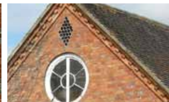
138 Berkshire orange brick with a variety of features including: blue headers and string course, buff detailing, diaper work and dentil and bottle work
