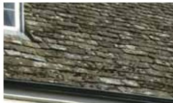
101 Traditional and modern replacement stone slates
