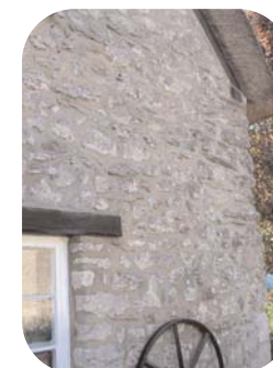
Inappropriate hard cement mortar
