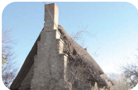
Stepped stone chimney stack 41 Leys Road
