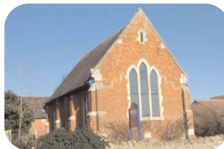
Red brick with limestone dressings, United Reform Church, Leys Road
