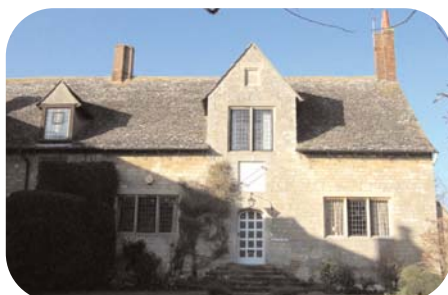
Stone dormer, sundial and datestone Cutts End House
