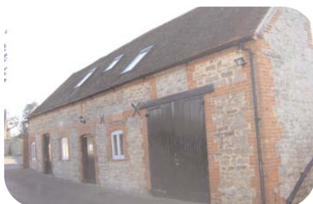
Clay tile, stone with brick dressings Stables, Archangel House (The Old Vicarage)
