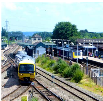
Didcot Station Source: Google Maps
