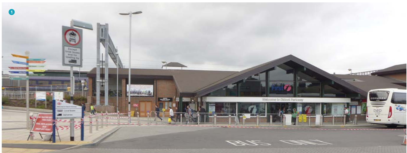
Existing: Didcot Station
