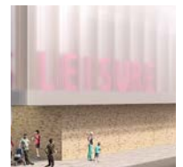
Didcot Leisure Centre
