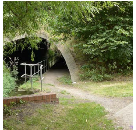
③ A4130 Underpass
