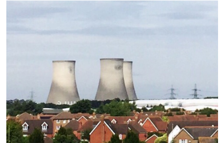
Construction of Didcot A power station's iconic cooling towers began in the 1960s
