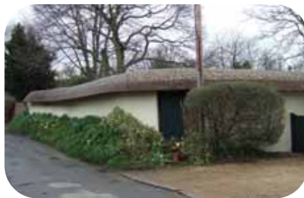
Thatch and Cob wall , Cat Street
