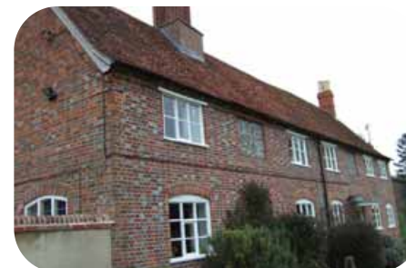
Diaper brickwork, Cozen's Farmhouse
