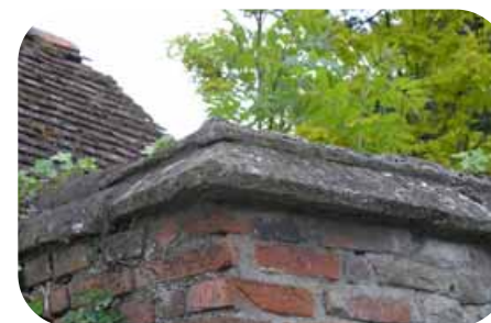
Stepped triangular capping, King's Manor
