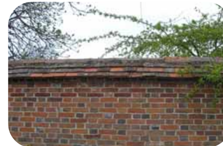
Stepped clay tile capping, Church Street
