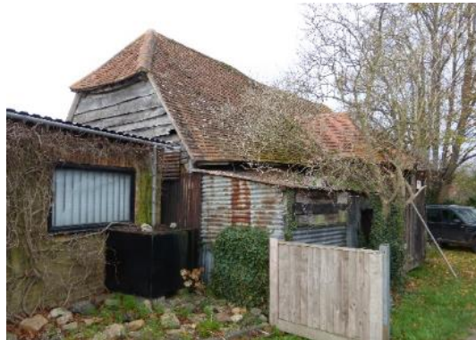
Barn 20m south east of Home Farm, School Lane Timber framed threshing barn with hipped clay tile roof and midstrey, wide waney edge elm boards & some repairs in corrugated iron
