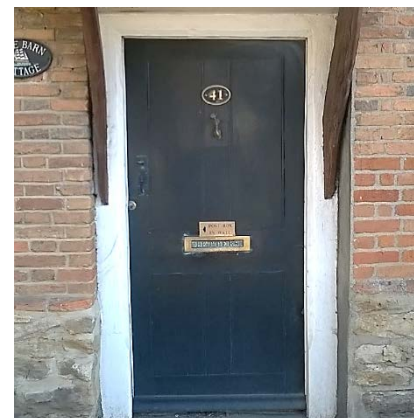
Tithe Barn Cottage: Timber panelled door in pegged oak door frame with chamfered head and jambs
