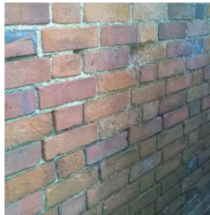
Typical brickwork in Flemish bond along boundary and lane walls
