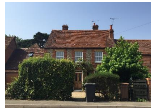
66 High Street C18, vitrified bricks laid in header arrangement with red brick quoining. Symmetrical frontage with 8/8 sash windows, stone lintels over
