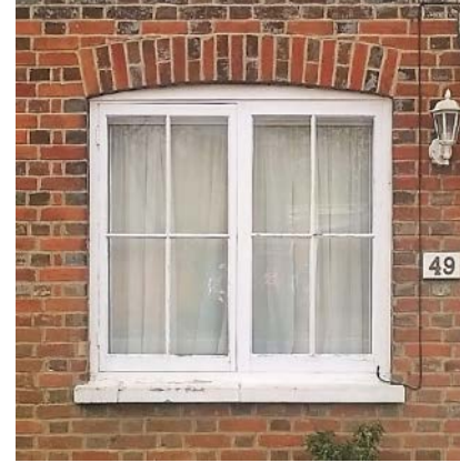
Side hung timber casement windows with brick arch window head
