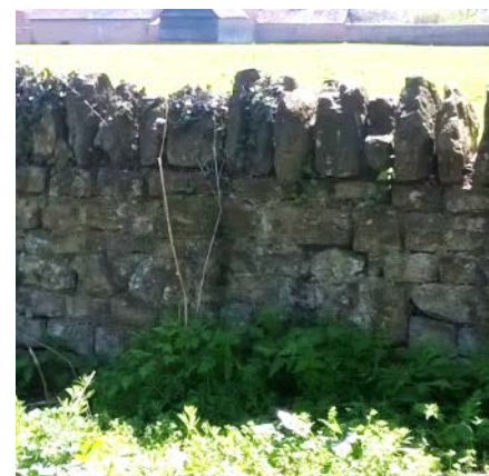
Stone boundary wall with stones laid on edge
