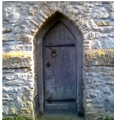
Church door with pointed arch wrought iron strap hinges and door furniture
