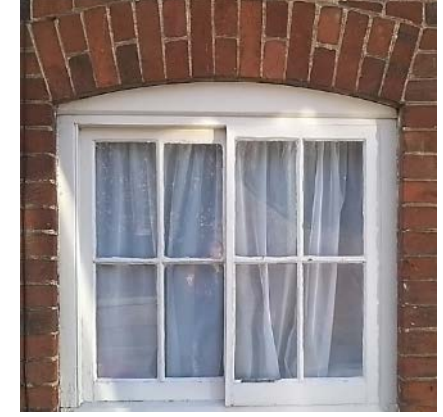
Horizontal sliding sashes with arched window head on cottages
