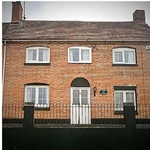
Fern Cottage: typical symmetrical façade of C19 date in Flemish bond brickwork
