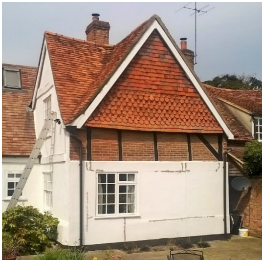
The Old Bakery: Clay tile hung gable with 'club and fishtail' detailing to shield the timber framed building from weathering and water ingress
