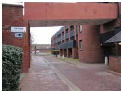
The Charter Area currently contains a multi-storey car park
