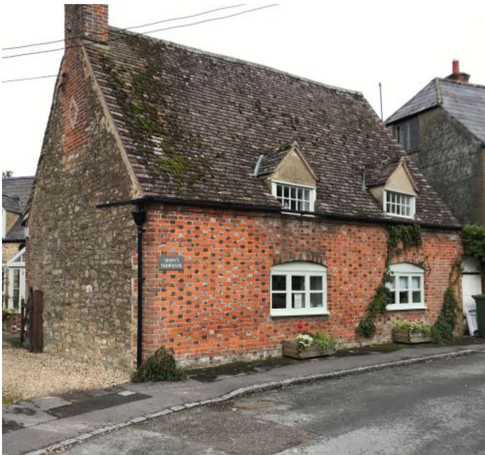
Fig 18. Green's Farm House 1650. Steep roof with narrow gable angle and tiny dormers, period 'diaper' brickwork, flush casement windows with segmental heads.
