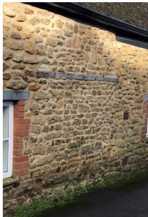
Fig 30. Clayton Villa c 1801. On-street structures now below street level and evidence of former openings onto street.
