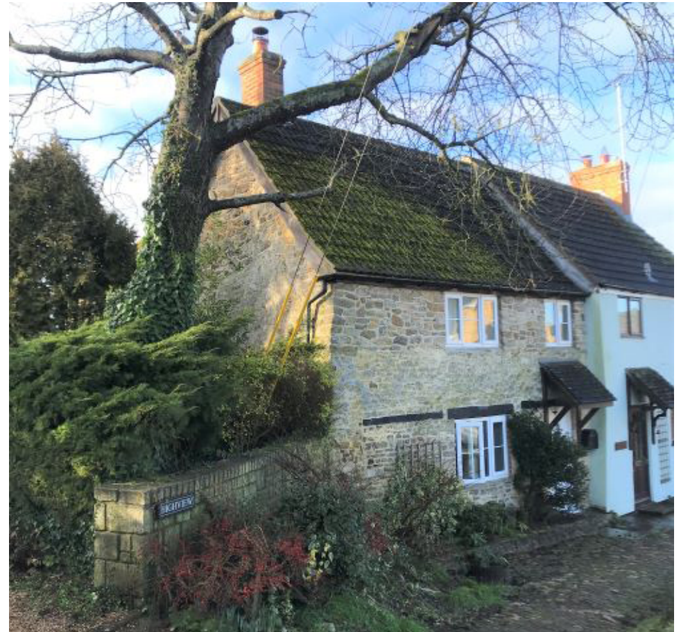
Pottinger Cottage, 1790 Irregularly coursed stone rubble with irregular stone quoins, some butter-pointing. More regular coursing at first floor level replaces a part-collapse when the earlier thatch was removed. Wooden lintels over four three- and two-light casement windows (another blocked). Brick chimney stack through ridge within house, thus several features earlier than date given.
