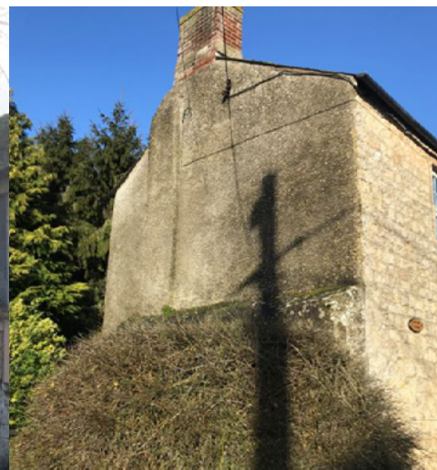
Fig 28. Box Tree Cottage, c 1890. Details: stone quoins, flat segmental window arches, lime wash remains, projecting bakery oven.
