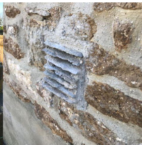
Fig 33. Warene House c 1820. A small vent of stone flags in lower wall on street.
