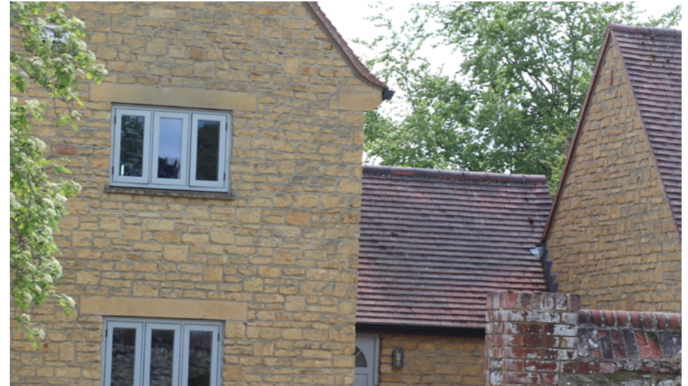
Fig 32. This modern house uses an inappropriate iron-rich Marlstone which has weathered to a mustard yellow colour.
