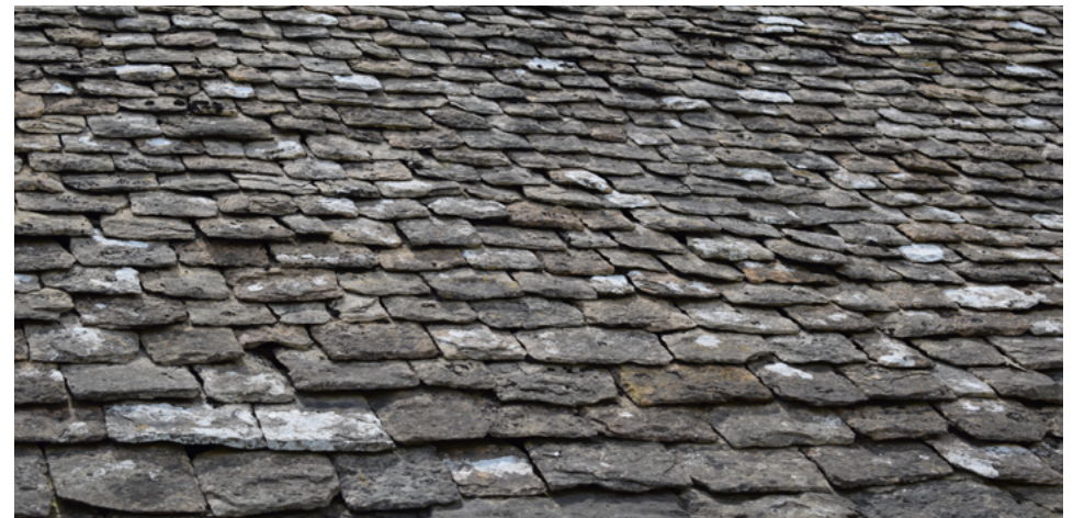
Fig 15. Stonesfield slate roof, near Stanford Manor House.
