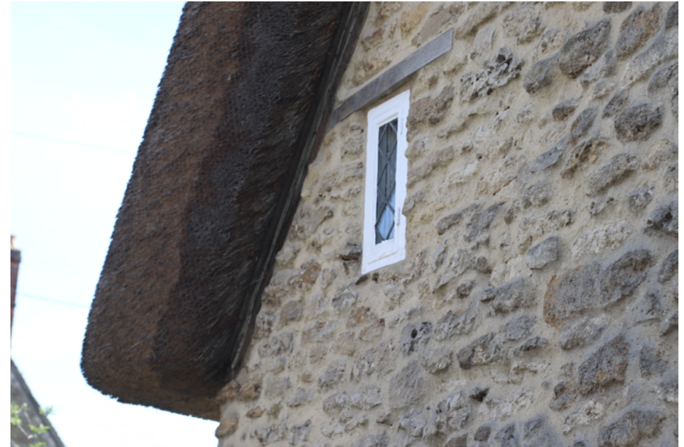
Fig 34. An example of good repointing using a lime based mortar, tamped back from the masonry face.
