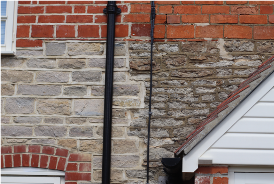
Fig 33. Examples of poor repointing. Soft mortars must be used with historic masonry and pointed flush, not weatherstruck or strap pointed as shown (left side is of a later extension “in-keeping”).
