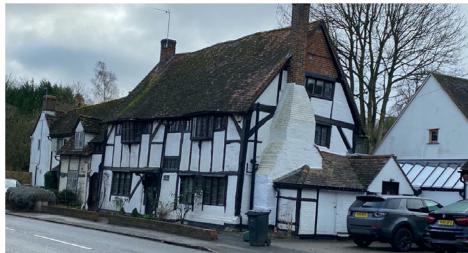
Fig 7. External chimney stack on The Dower House, London Road (listed as Double Doors)
