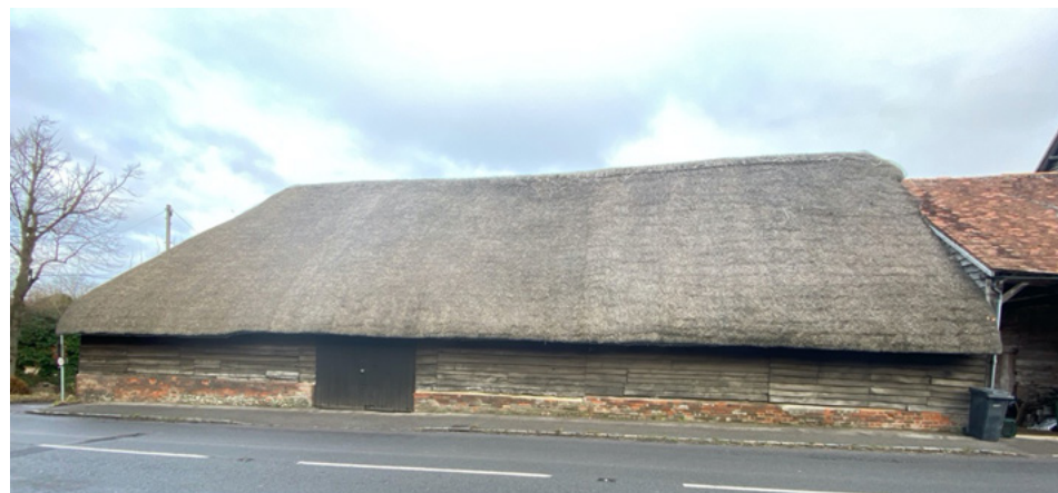
Fig 39. Barn at Great Tree Farm with weatherboarding and thatched roof
