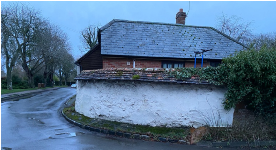
Fig 28. Tile-capped wall at the junction of Westbrook Street and Church End
