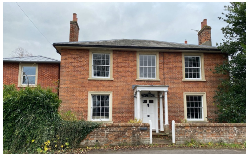
Fig 26. Curtoys, Westbrook Street, a typical early nineteenth-century house with two full storeys, hipped slate roof, double-hung sash windows and Doric open porch
