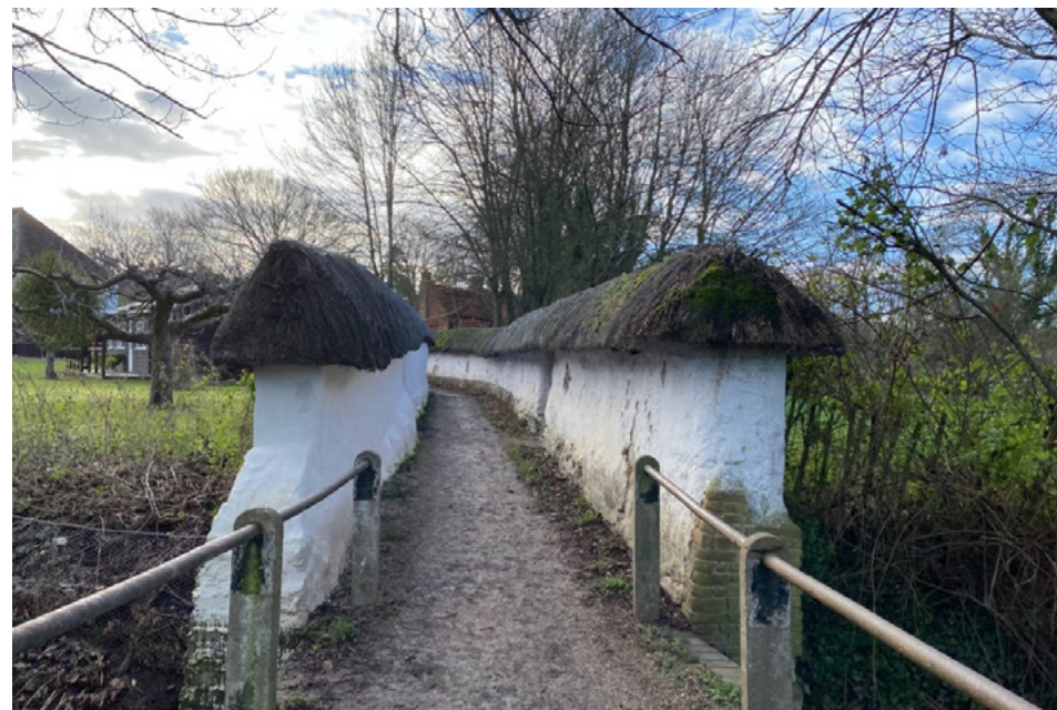
Fig 17. Cob walls with thatch capping lining footpath near Chapel Lane
