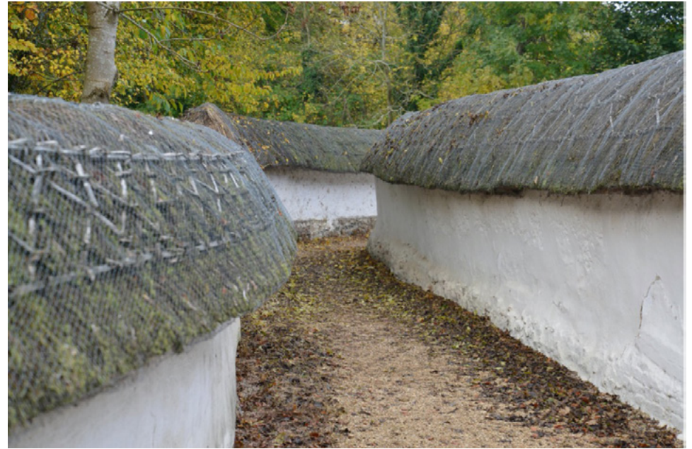
Fig 1. Cob walls with thatched cap defining ancient pathway
