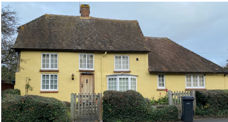
Fig 8. Ayres Cottage, London Road, showing a central stack in line with a central entrance, indicating a lobby entry plan
