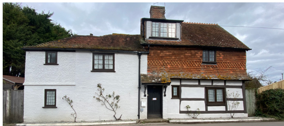
Bridus House, South Street
