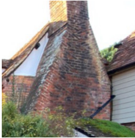
Fig 21. Chimney stack at Cherry Patch
