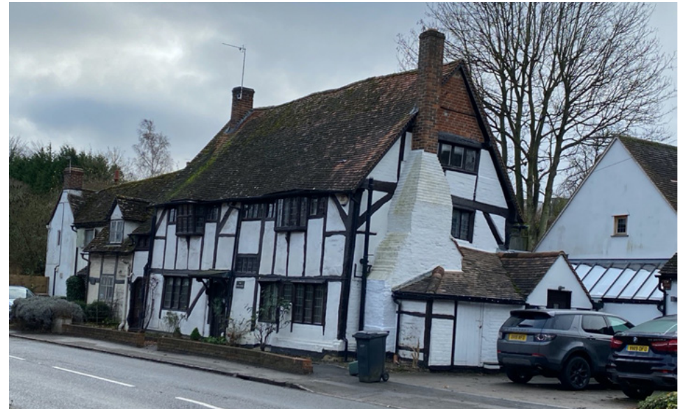
Fig 40. Dower House, showing external stack, early windows of varying dates
