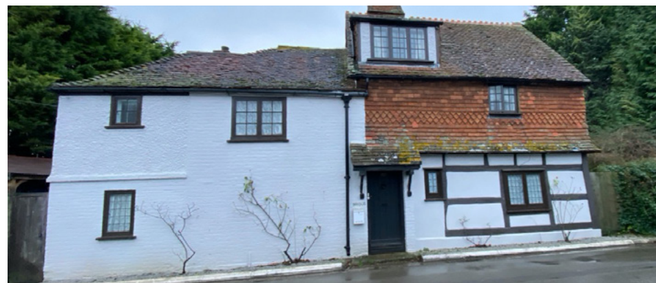
Fig 35. Bridus House, a multiphase house showing alterations over time in a range of materials
