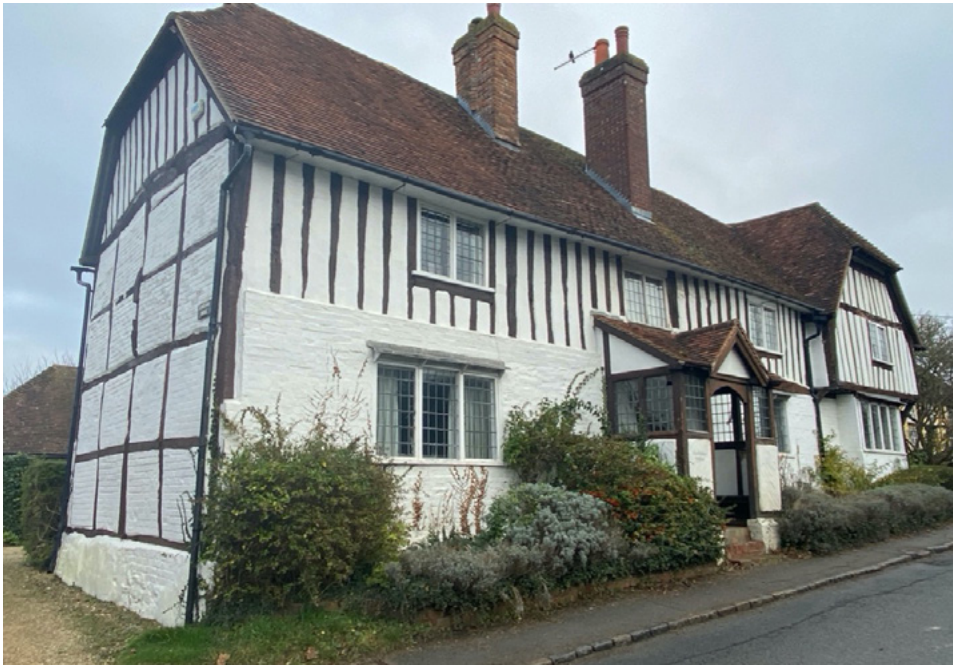
Fig 3. Close studding on the front elevation and upper gable of Corrydon House. The less visually prominent gable is constructed on the less impressive small square panels
