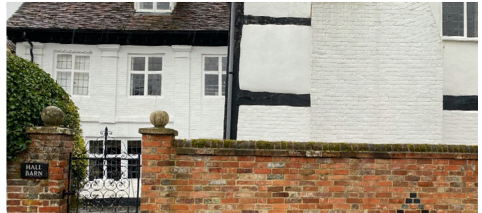
Fig 23. Hall Barn showing Doric pilaster in brick. Also visible is the external stack of the earlier timber-framed wing
