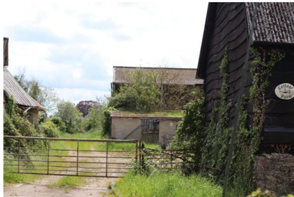
Fig 36. Cottage Farm overgrown and in a state of neglect
