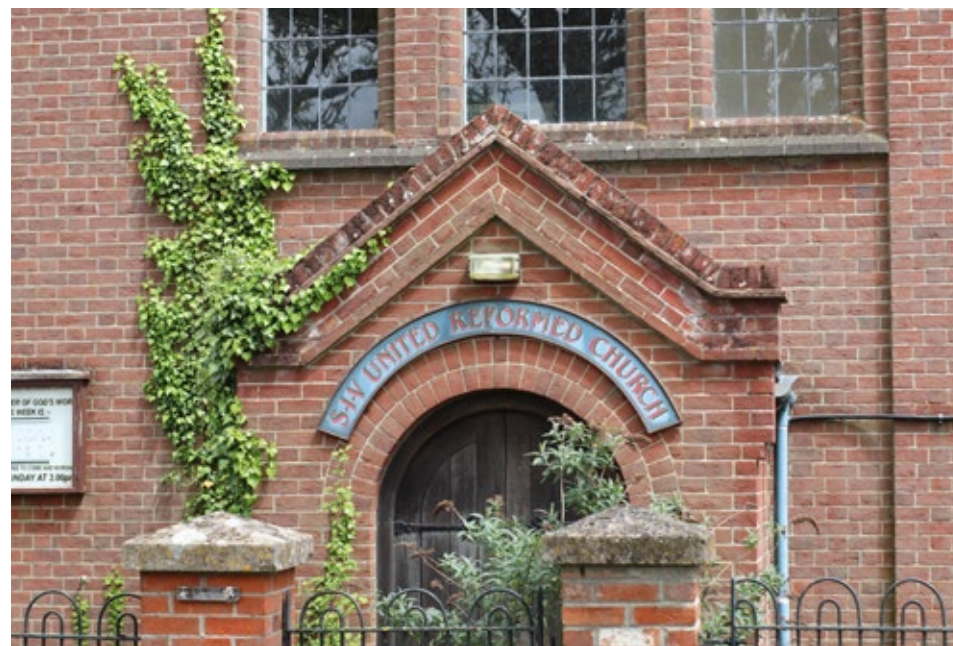
Fig 35. The presently empty United Reformed Church on Chapel Road
