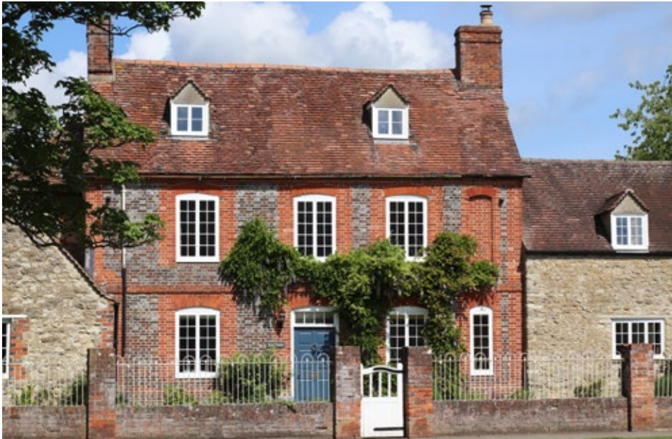
Fig 6. Bear House; example of an earlier house refronted in the early Georgian period
