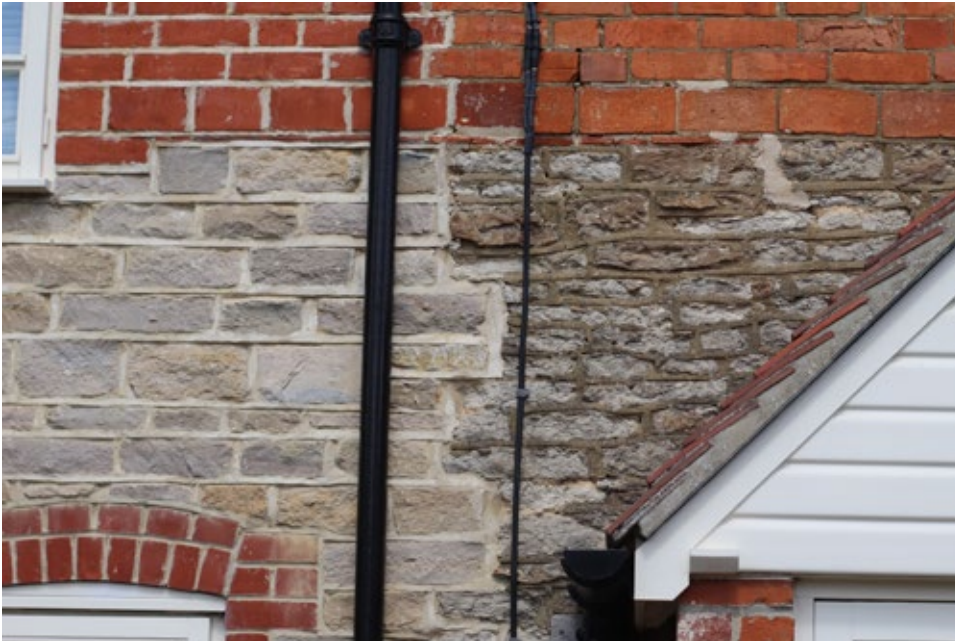
Fig 33. Examples of poor repointing. Soft mortars must be used with historic masonry and pointed flush, not weatherstruck or strap pointed as shown (left side is a later extension “in-keeping”)
