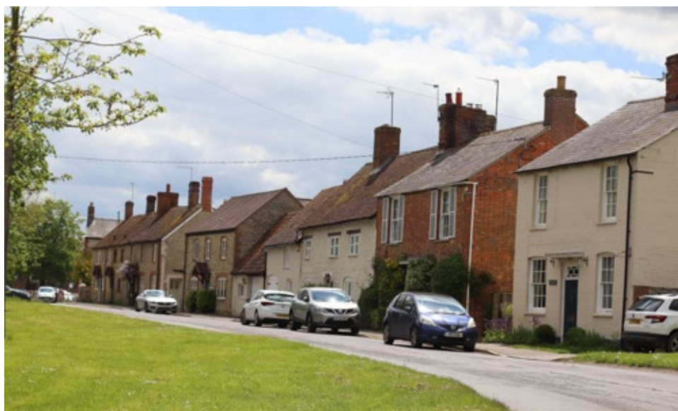
Fig 7. Labourers' housing on Chapel Road.
