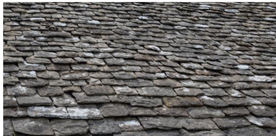
Fig 15. Stonesfield slate roof, near Stanford Manor House
