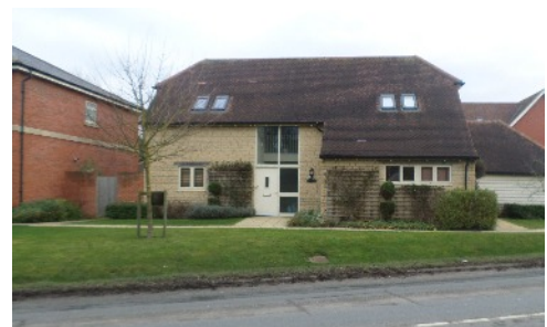
Figure 64: Cotswold Stone is not a material found within the village historically
