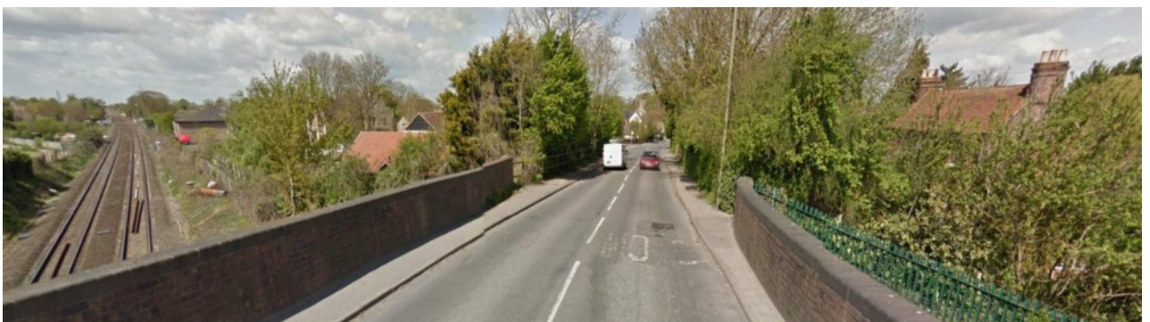
Figure 37: View westward along the railway line
