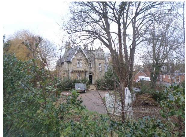
Figure 32: Grade II Listed Brook House
