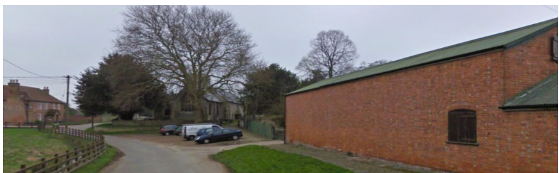
Figure 47: View from the junction of The Causeway, Mill Street and Church Lane to the Church and Manor Farm
