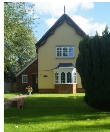
Figure 78: Milton Lane contains a significant number of historic and listed buildings. Although constructed in the early 1990s, this dwelling successfully draws on a number of references to its historic setting
