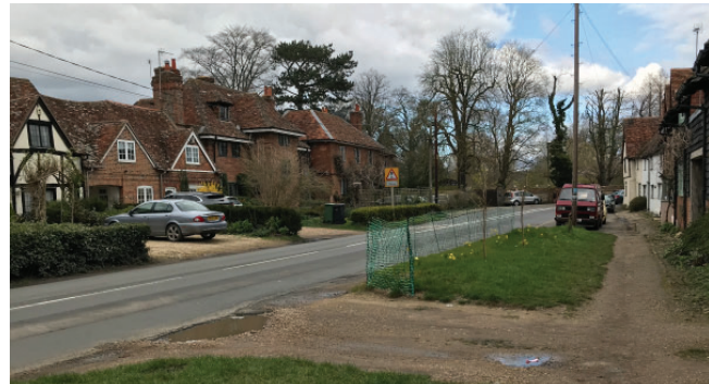
Unmade paths without kerbs are part of the character of the village
