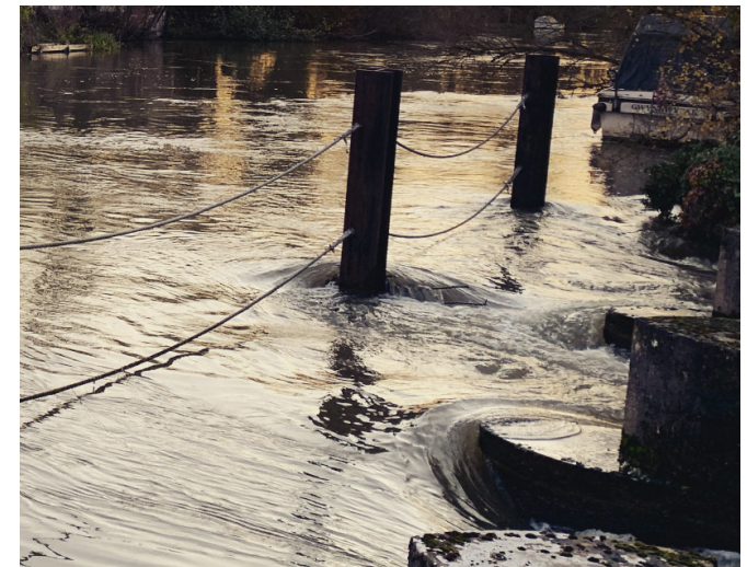
The Thames in flood north of the village edge, with sluices open to expand channel capacity to the north
