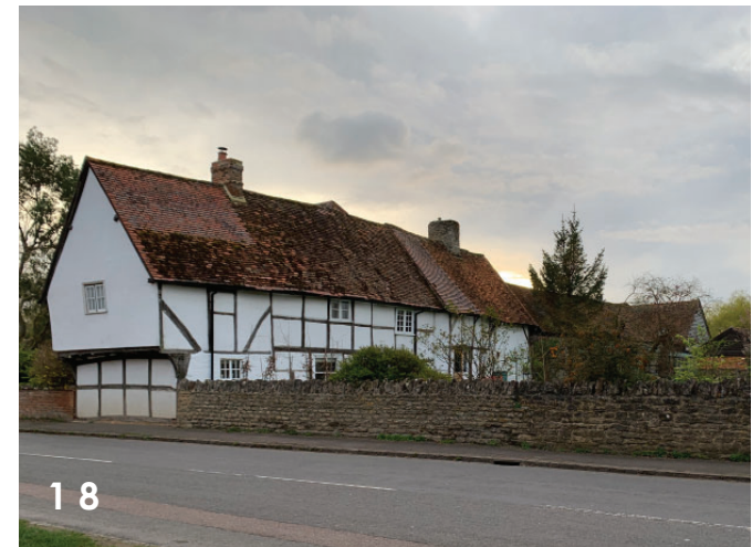
18 58 High Street, Southfield Farm, looking south opposite Lady Place
