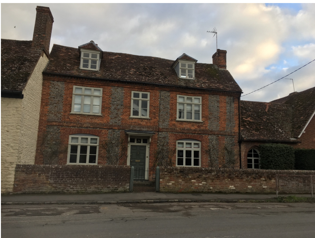
Figure 21. There are several examples of blue-grey bricks used with red brick for decorative effect (February 2019)
