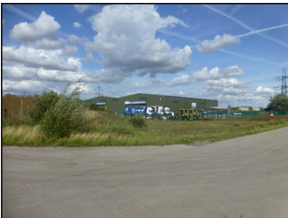
View north east from 373/10, by the access road to the composting area, showing the FCC Environment recycling plant.
