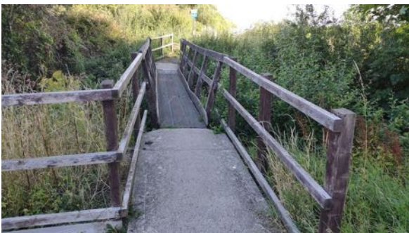
View north, of the old bridge over Moor Ditch, prior to its demolition 2020. This bridge was used in lieu of the older Moor Ditch bridge at the end of Milton's FP 299/1 and FP 299/2.
