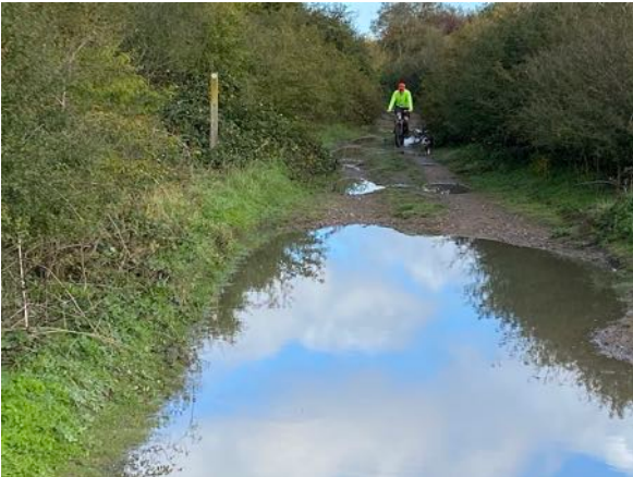
View of 373/10, Old Wallingford Way, north showing the section that floods after any rainfall. There are ditches on both sides but the grips are not maintained so the water does not drain away.
