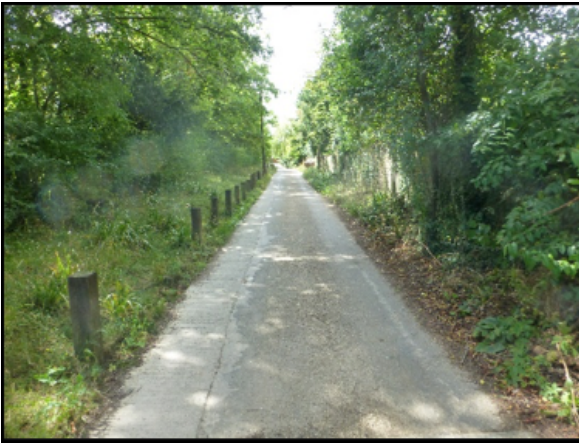
View south along the concrete roadway servicing the housing and leading to the lakes on the left.
