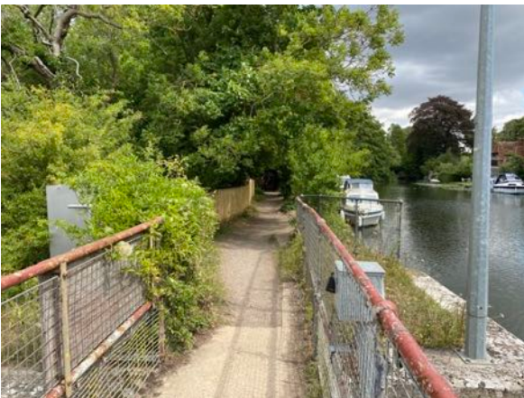
View downstream from the second weir. Low level fence to the spit of land belonging to Mill House.
