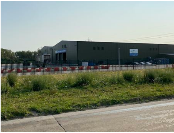
BOATs 373/9 and 373/10, Hobbyhorse Lane and Old Wallingford Way, meet at the FCC Environment recycling plant.
