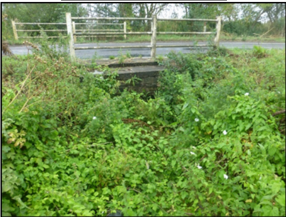
View from the end of 373/12 where the designated Right of Way meets the north end of 373/31 and Appleford Rd, B4016. A large diameter black pipe crosses the path and is a tripping hazard.
