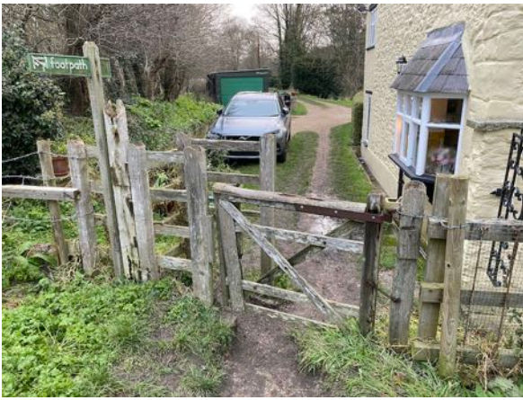
View back, north, across Kissing Gate next to Ginge Cottage. The kissing gate is very small and in poor repair. Note the old style finger post pointing along FP 373/16 and showing a stile, which no longer exists.
