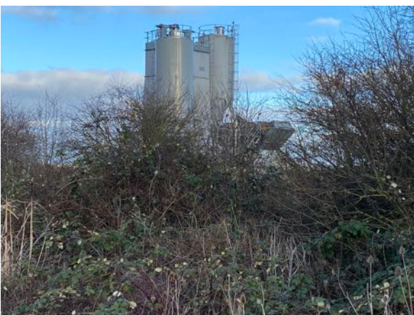
View east, of the aggregate washing and grading plant belonging to Hanson.
