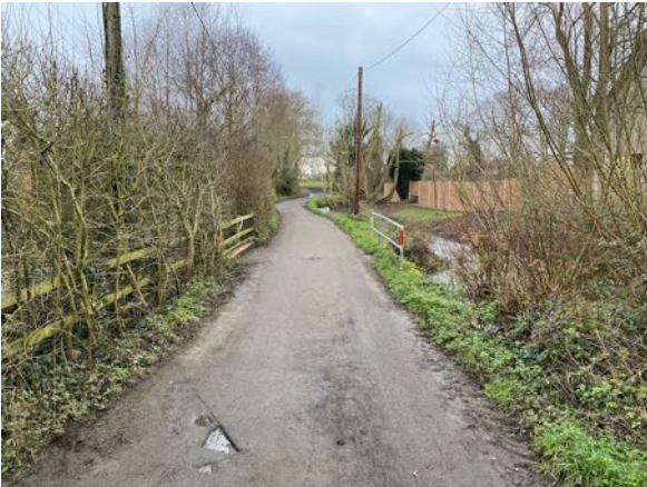
Bridge over Ginge Brook on 373/26.
