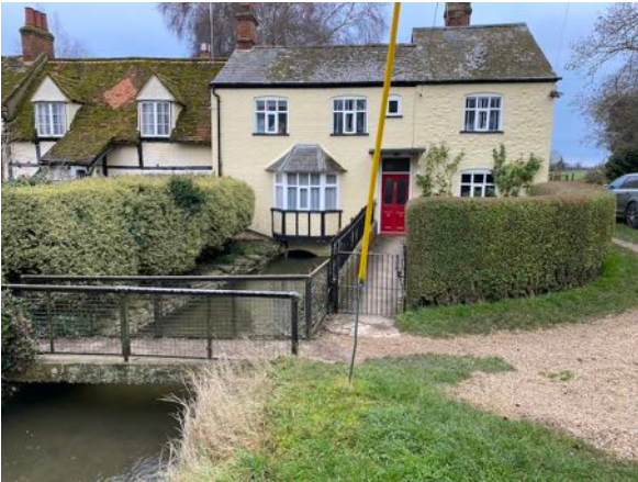
View looking south, along FP 373/14 junction with FP 373/13, over the bridge in front of the Mill House, No. 3 Ginge Brook.
