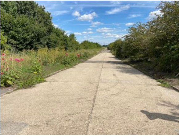
View north, along the Spine Road, a service road belonging to the power station site.
