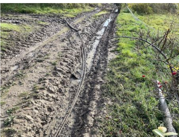
Hobbyhorse Lane, BOAT 373/9 is criss-crossed with large and small bore pipes to do with gas extraction from the landfill site to the south, these have now, 2020, been buried.
