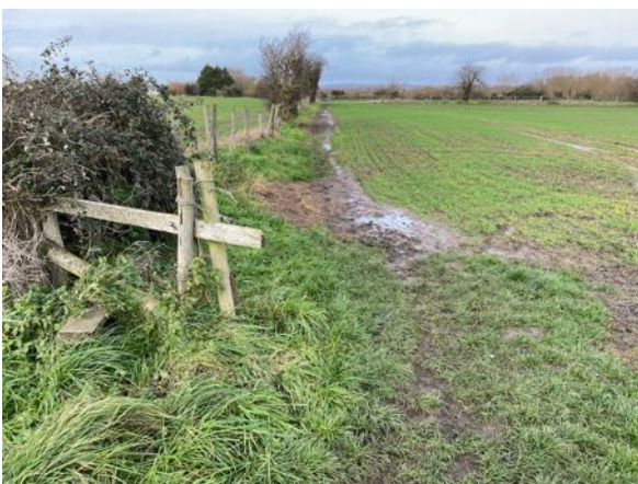
View north, showing the broken stile and FP 373/15, toward Drayton Road.
