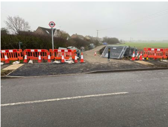
Milton's FP 299/1 and the shared use Cycle Track starts from the end of Milton Road and goes south to Milton Park, past the back of the houses on Tyrrell's Way; some have gates on to this path. This view shows the new signage and pavement crossover, installed January 2021.
