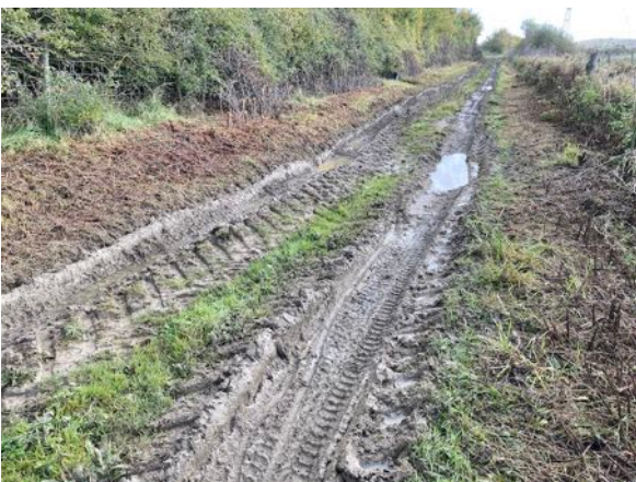
View east along Hobbyhorse Lane, BOAT 373/9. The monitoring points for the landfill are dotted along the PROW and the damage is largely due to the vehicles used to access the monitoring points resulting in the deep ruts.
