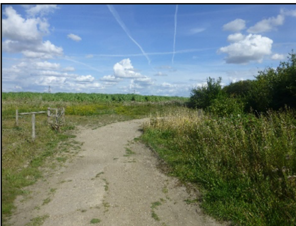
The Byway, 373/10, doglegs right then left and deteriorates markedly. Many people continue straight on, east, to a track across the field, which runs parallel to the Byway and is in slightly better condition. There is also a path to the left, north, between the fields.
