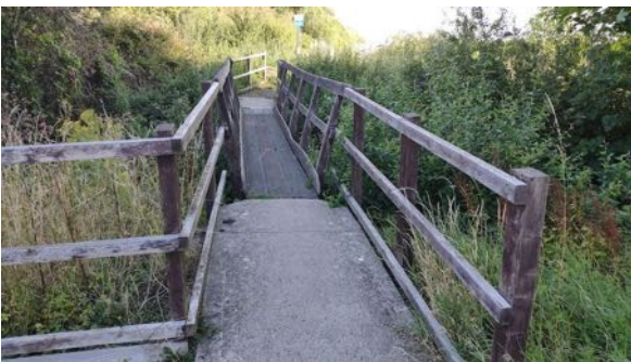
View north, of the old bridge over Moor Ditch, prior to its demolition 2020. This bridge was used in lieu of the older Moor Ditch bridge at the end of Milton's FP 299/1 and FP 299/2.
