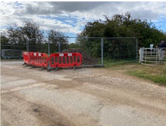
View SE from Oday Hill, 373/22, showing the kissing gate to FP 373/32 and continuation of Bridleway 373/18, Peep-o-day Lane, to the left. Fencing remaining from the resurfacing work to 373/18, July 2020.
