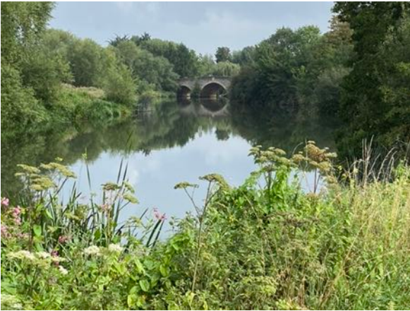
One of several nice views of Sutton Bridge.
