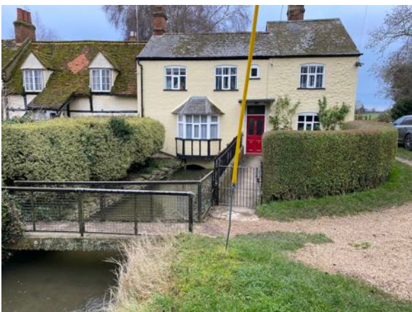
View looking south, along FP 373/14 junction with FP 373/13, over the bridge in front of the Mill House, No. 3 Ginge Brook.
