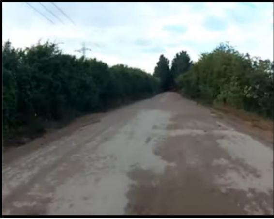
This section of Peep-o-day Lane is a wide gravel quarry road. Dusty when dry, muddy when wet.
