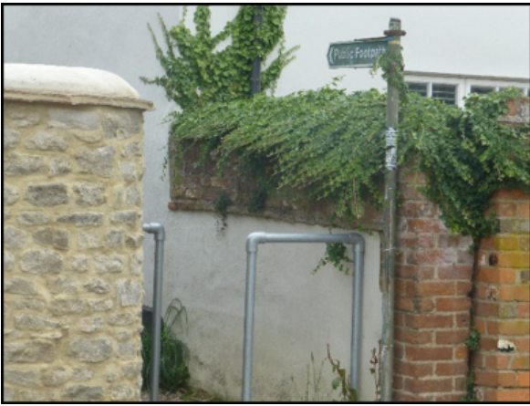
Finger post and offset Barrier at High St entrance to path
