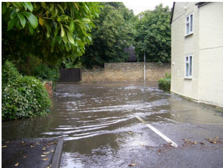
Figure 7.4 Brook Street/Chapel Lane Flooding
