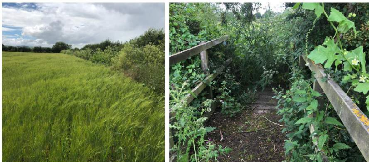
Figure 21. Examples of neglected footpaths north of East Challow. Left image, unmarked path through cereal field. Right image, overgrown bridge crossing ditch, blocked by vegetation.
