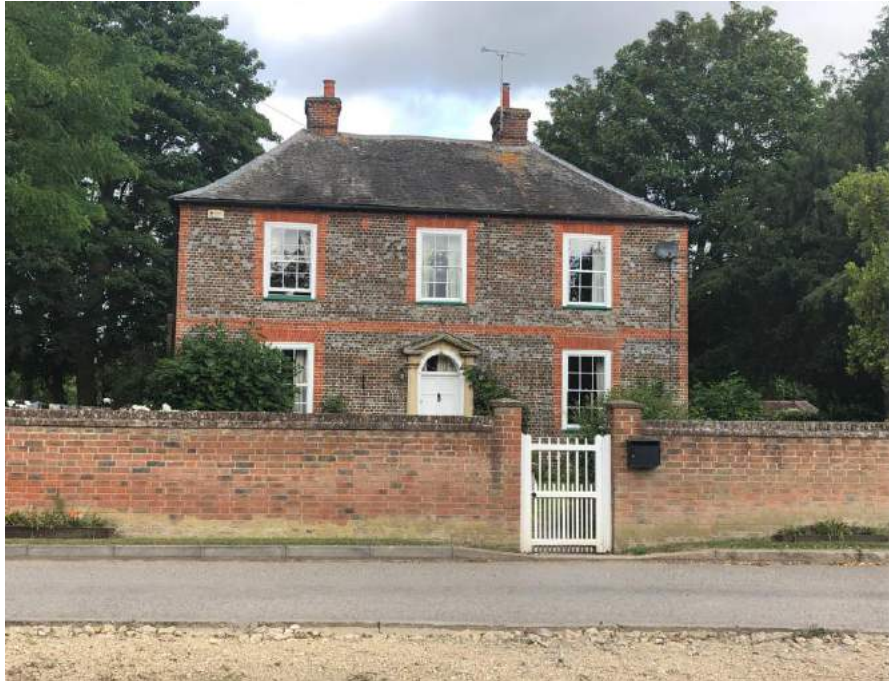
Figure 37. Listed building 18 th century farmhouse.
